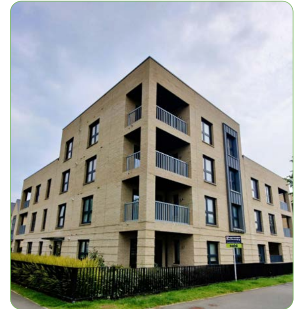
Inset balconies at Alconbury Weald provide shade and improved privacy
