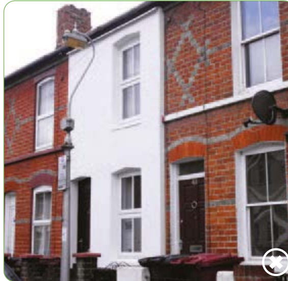
An insensitive external wall insulation application which damages the beauty and character of the street (Source: Planning Responsible Retrofit of Traditional Buildings - Sustainable Traditional buildings Alliance )
