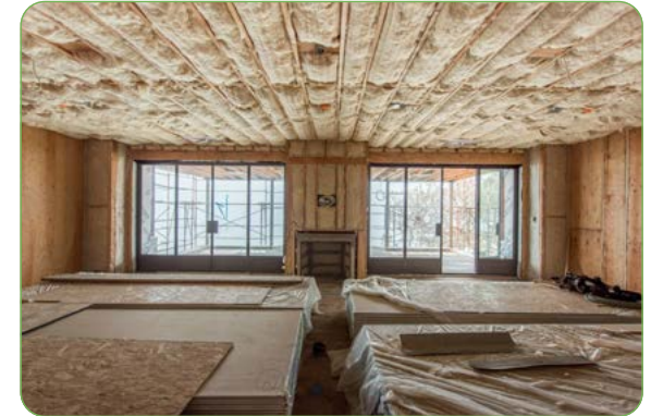
Natural Sheep's Wool insulation (source: https://havelockwool.com )
