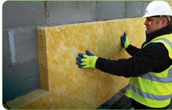
Glass wool insulation batts being installed in a full-fill cavity wall (source: www.selfbuildanddesign.com )
