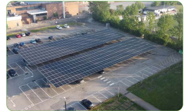
Solar Car Barns used at One Leisure St Ives
